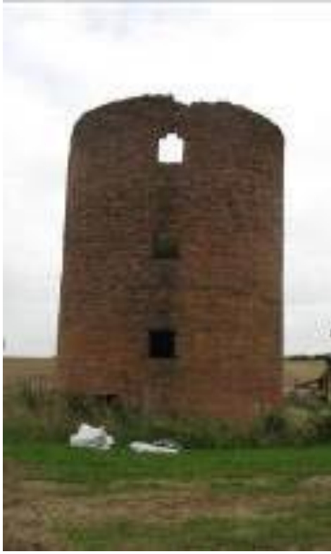
Old Grain Silo Swangleys Lane
